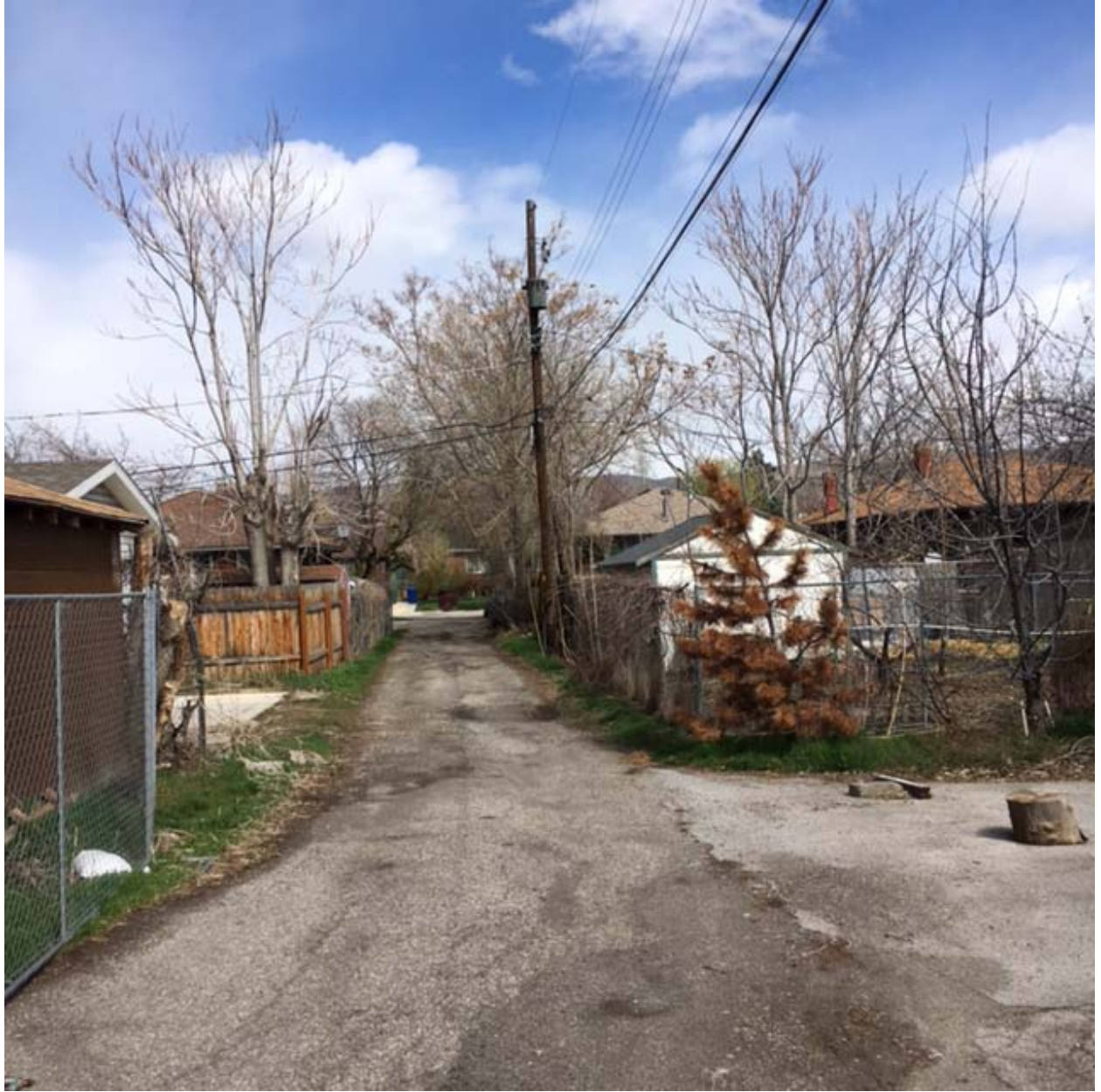
This is a photograph looking north along the existing alley.
